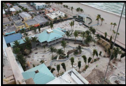
Pool and surrounding area progress
