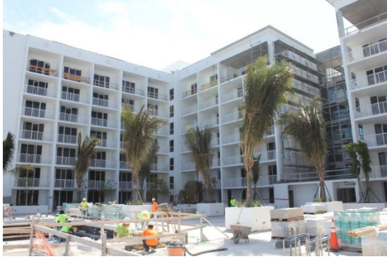
Figure 1: Progress on Level 11 pool deck
