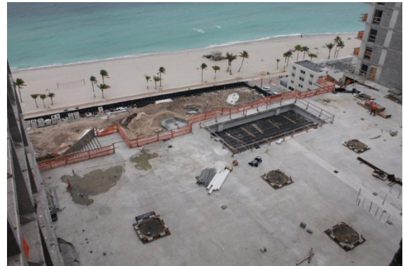
Figure 2: Deck sealed on level 11 pool deck
