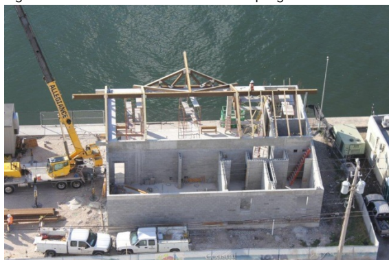
Figure 1: Five O'clock Somewhere Bar progress on intracoastal
