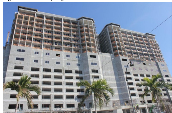
Figure 2: Stucco progress as seen from A1A
