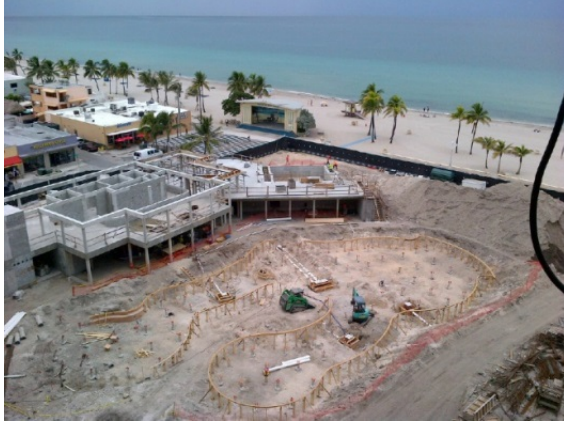
Figure 1: View of pool layout and waverider deck progress
