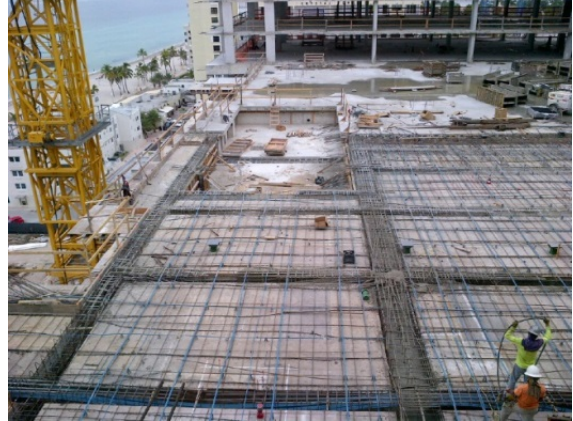
Figure 2: Concrete beam and Pool progress on Level 11 deck
