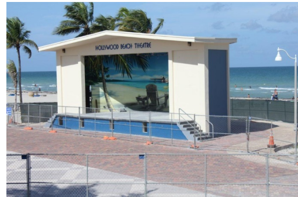
Beach Theatre has been re-vamped
