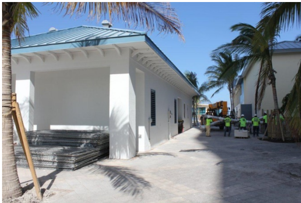
Johnson Street facilities and pavers
